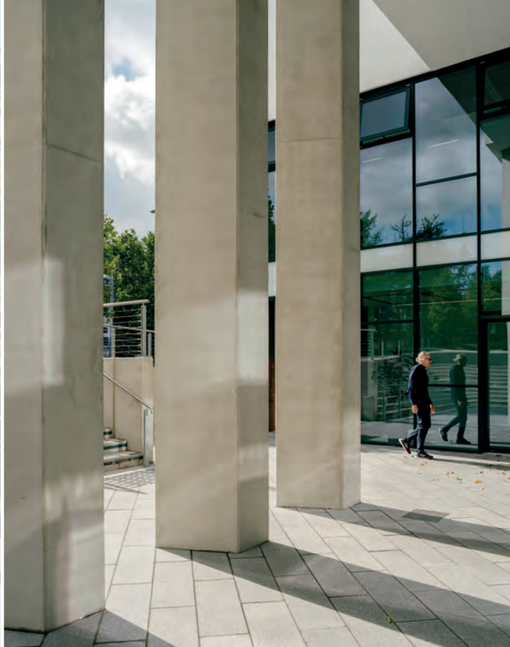
Above: Entrance portico formed with parallelogram-shaped columns.
